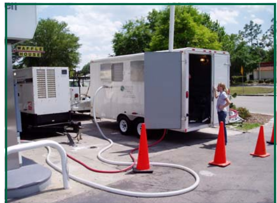
Picture 2 Plumbing Pilot Test Equipment
