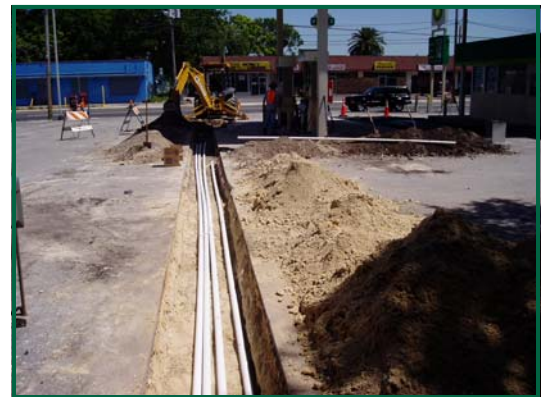
Picture 3 Piping Trench Connecting Recovery Wells to Treatment System
