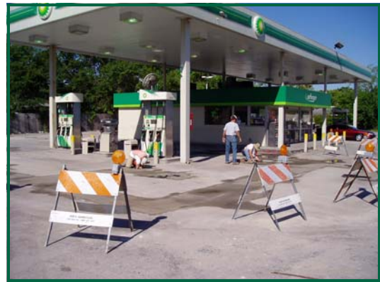
Picture 6 Concrete Resurfacing of Piping Trenches
