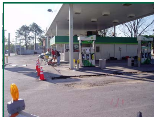
Picture 2 Trench Layout For Remedial Piping
