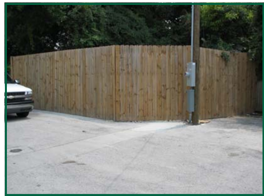
Picture 8 Remedial System Compound
