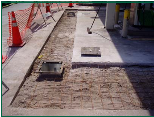
Picture 5 Recovery Well Vault Installation
